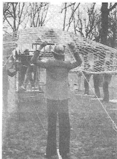
4. Draping the grid over tempor- ary support
