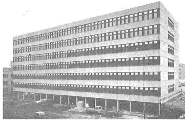
Fig. 5: Multi-purpose building at Technical University of Aachen
